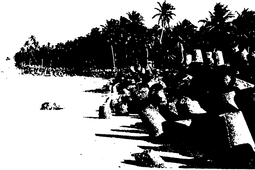
Figure 9. Erosion of the sea shore at Kavaratti atoll after coral quarrying. The tripods check further erosion
