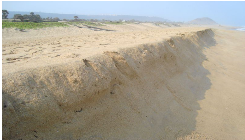
Fig.7. Beach erosion (viewed from south to north) observed during September at station:1. (Northern most profile)
